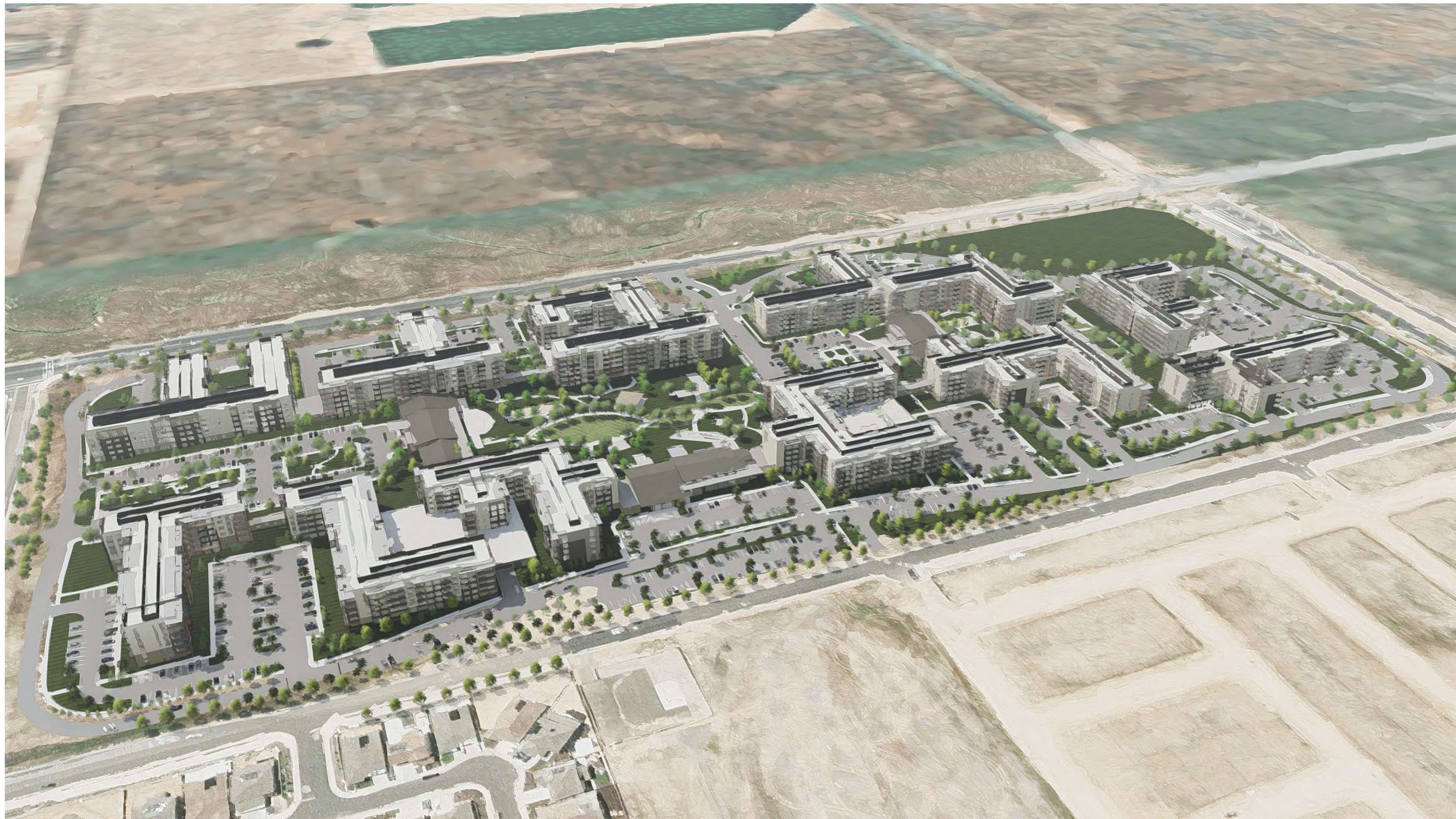
AERIAL VIEW FROM NORTH
